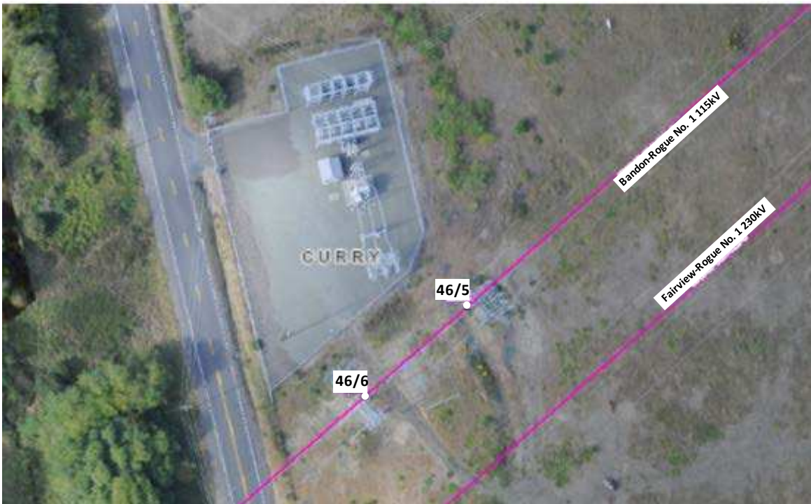
Figure 3: Aerial View of the 46/5 and 46/6 Structures at the Geisel Monument Tap
